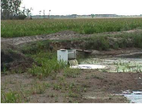
36-4 Water Control Structure
