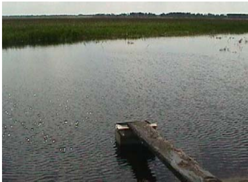
36-3 Water Control Structure
