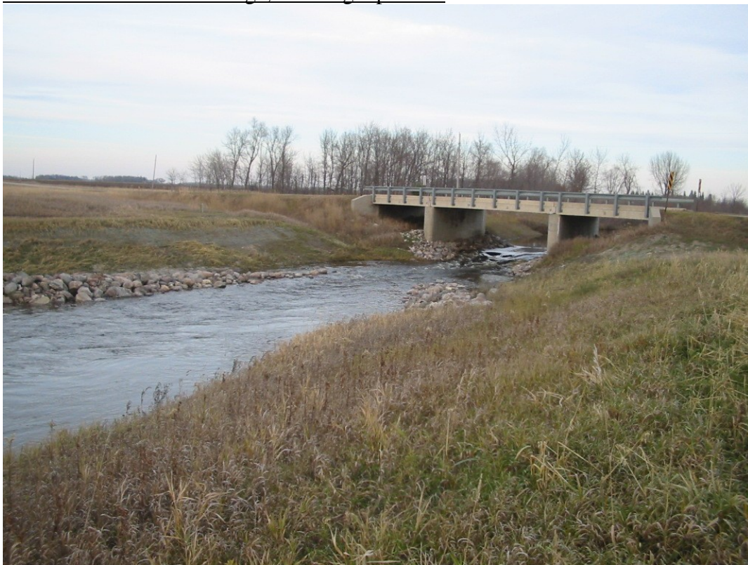
Cross-Vane Weir and Bridge, Looking Upstream
