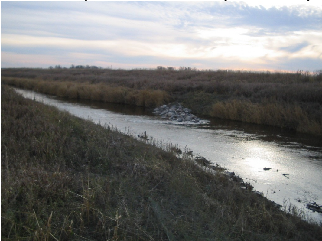
Stream Barb Directing Flow Toward Mid-Channel During November 2004 High Flow
