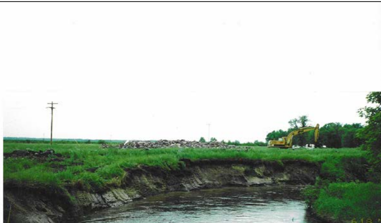
Site A Before Construction, Bank Slumping
