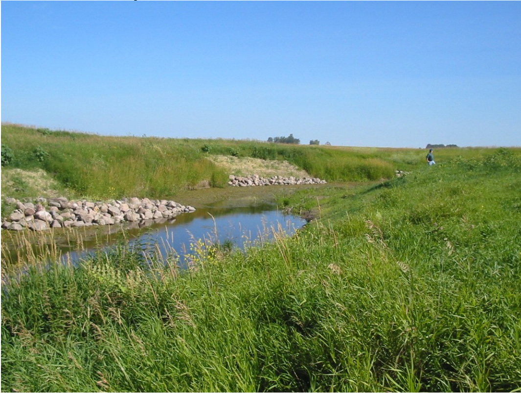
Stream Barb Directing Flow Toward Mid-Channel During November 2004 High Flow
