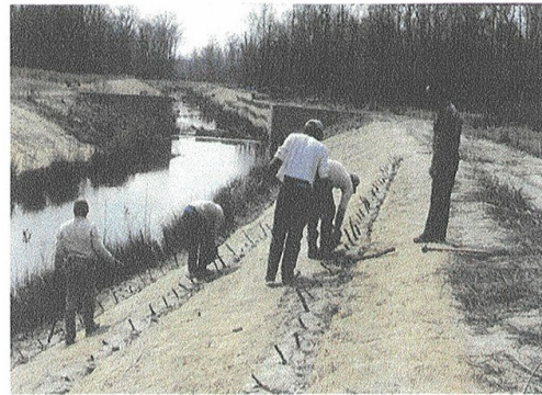
Installing live stakes in live fascine system
