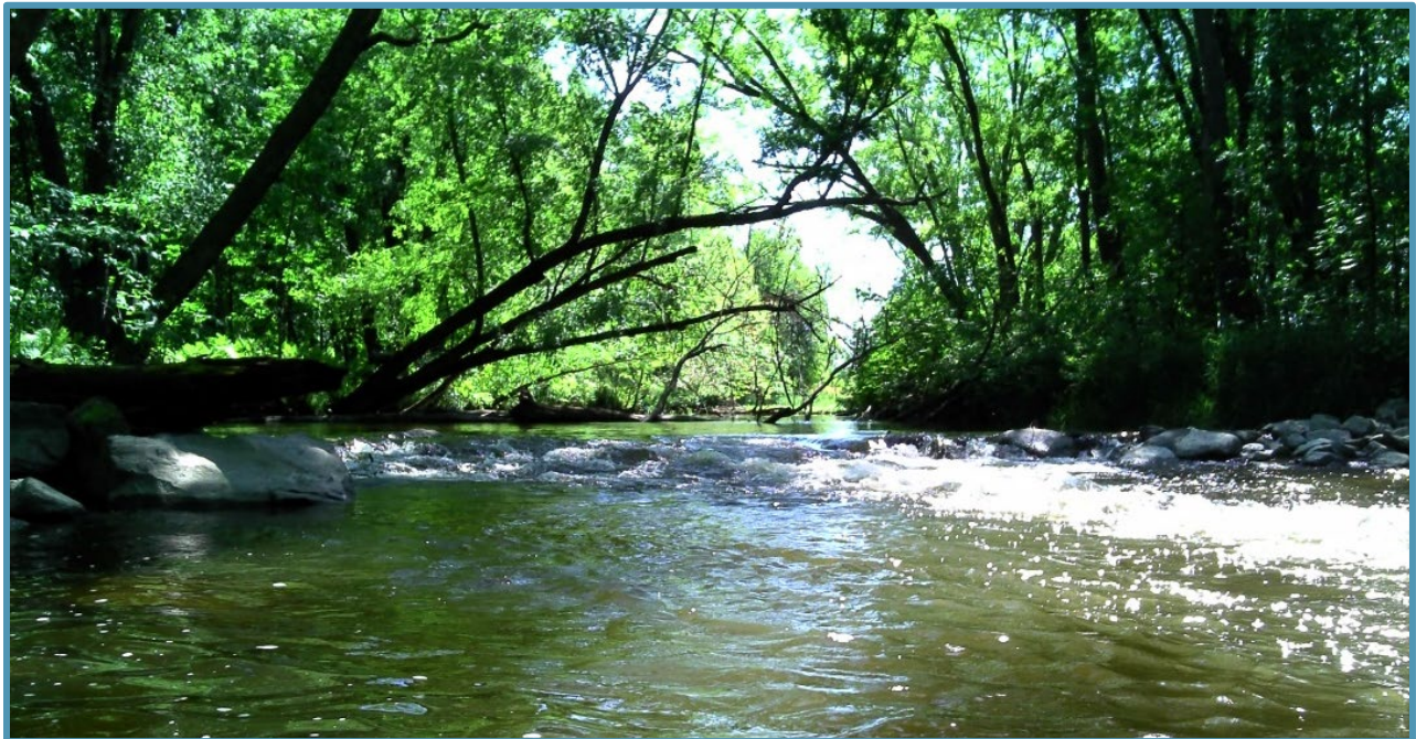
Figure 3.5. Rock riffle grade stabilization structure on the Clearwater River, installed as part of the Clearwater River Stream Bank Stabilization and Revitalization Project (RLWD).
